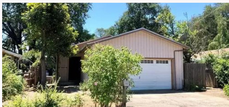
2nd Street Annex, Lakeport
